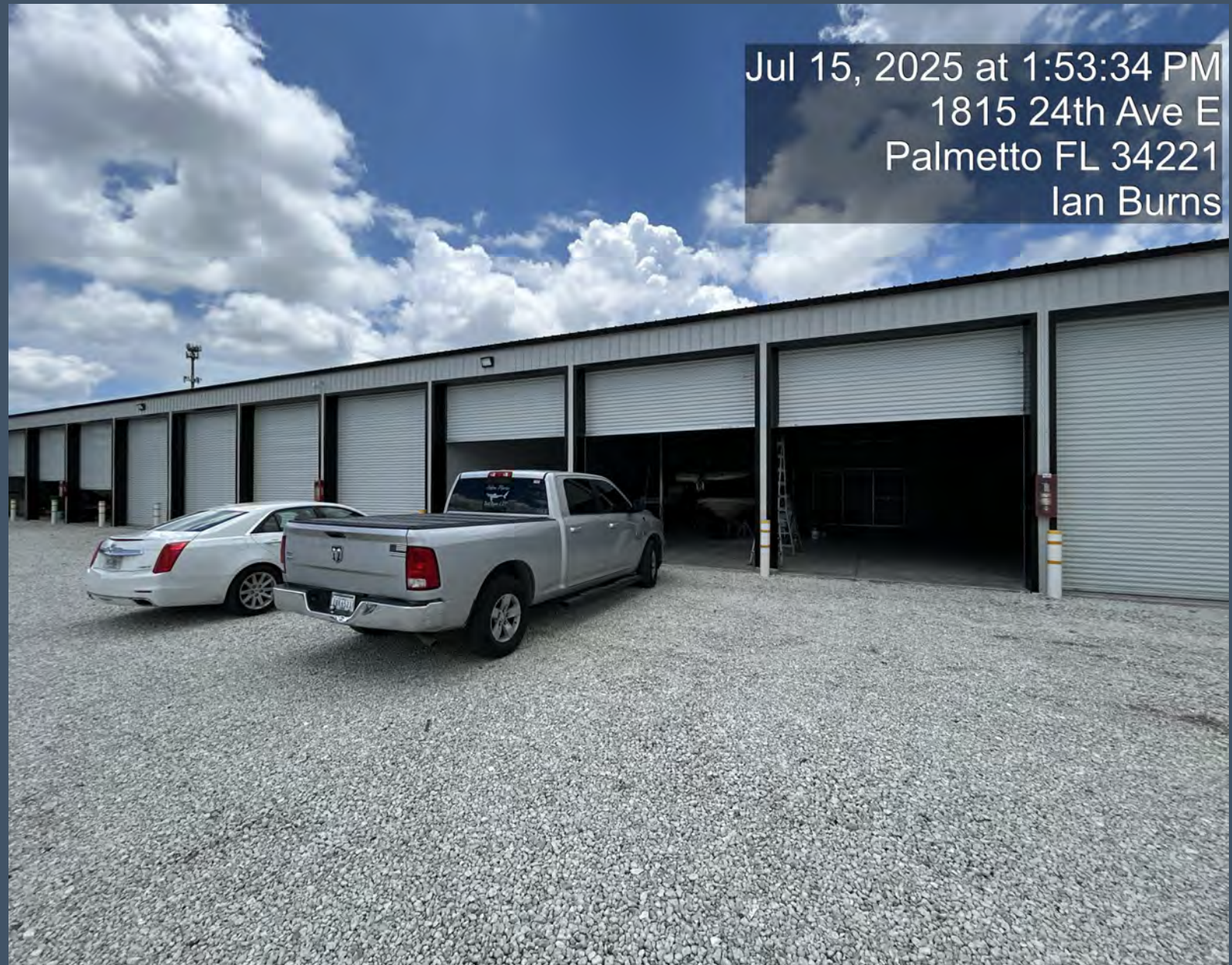
Photo depicts the bay doors that were installed
